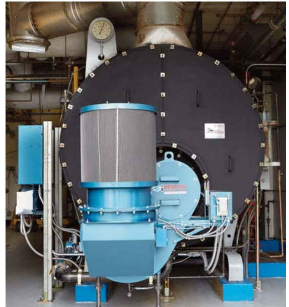
HDFX BURNER INSTALLATION
